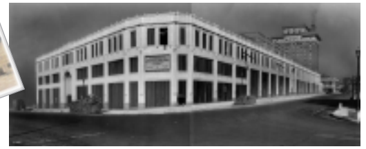
The Grove Arcade nears completion. Photograph by Herbert Pelton, 1927. Courtesy of North Carolina Collection, Pack Memorial Public Library, Asheville, North Carolina.
